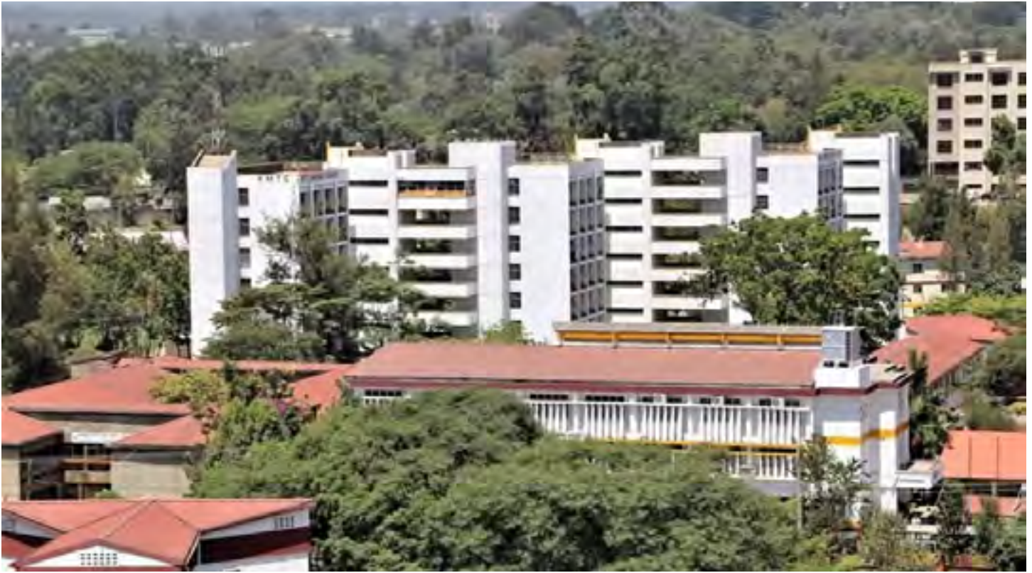
Aerial view of KMTC Nairobi Campus
